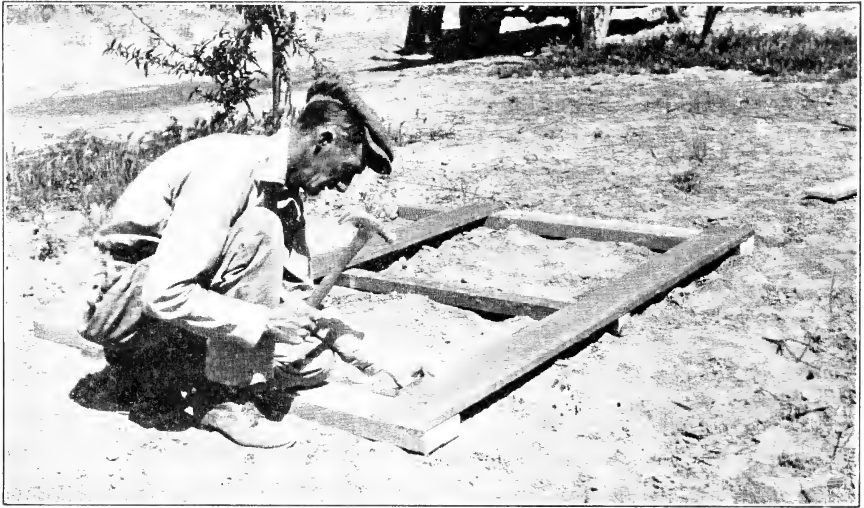
Fig. 6—Squaring up and starting the side-wall form.
